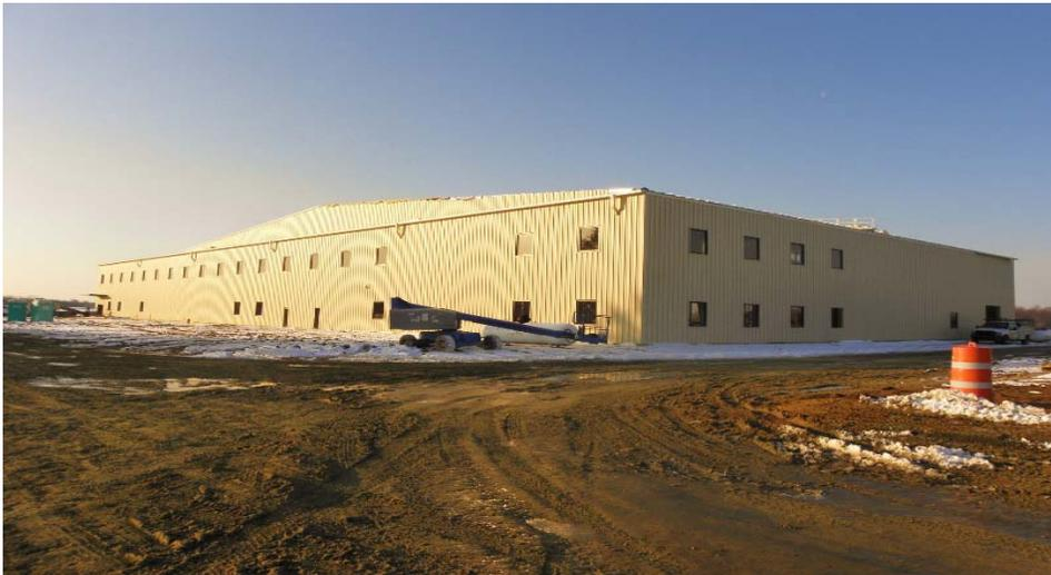
Summit Aviation's expansion is well underway. This new hangar is already 50-percent complete with the concrete floor being poured and wall structures in place.
